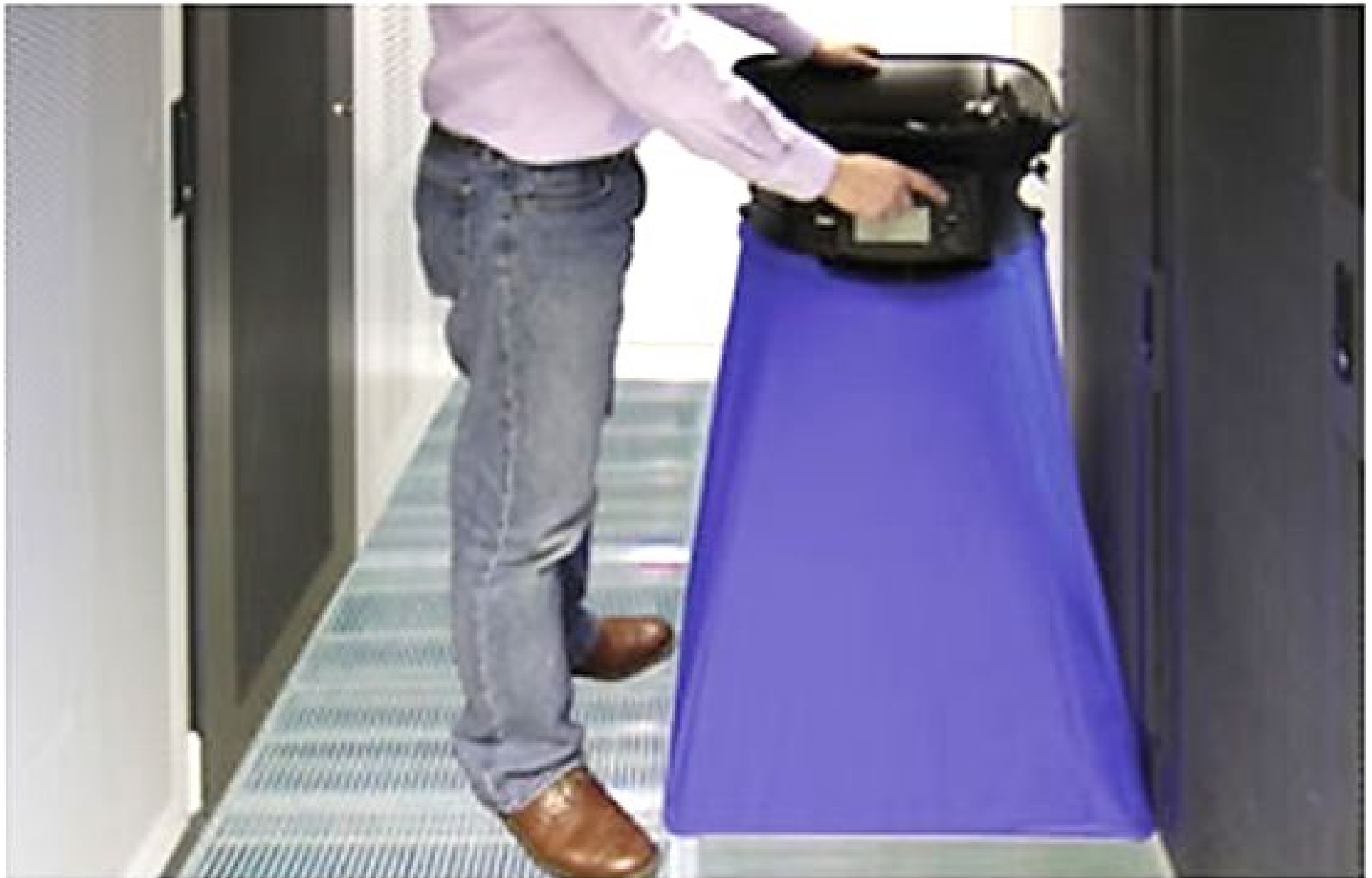
Perforated Floor Tile Flow Rate Analysis
